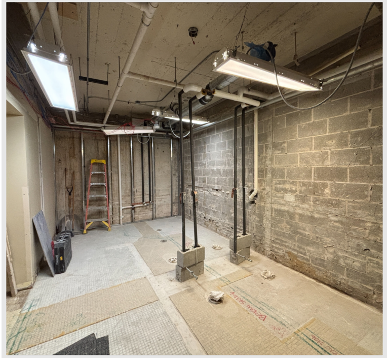
Selective demolition nearly complete in the Lower-Level Restrooms. Layout and prep is complete for concrete saw-cutting to begin!
